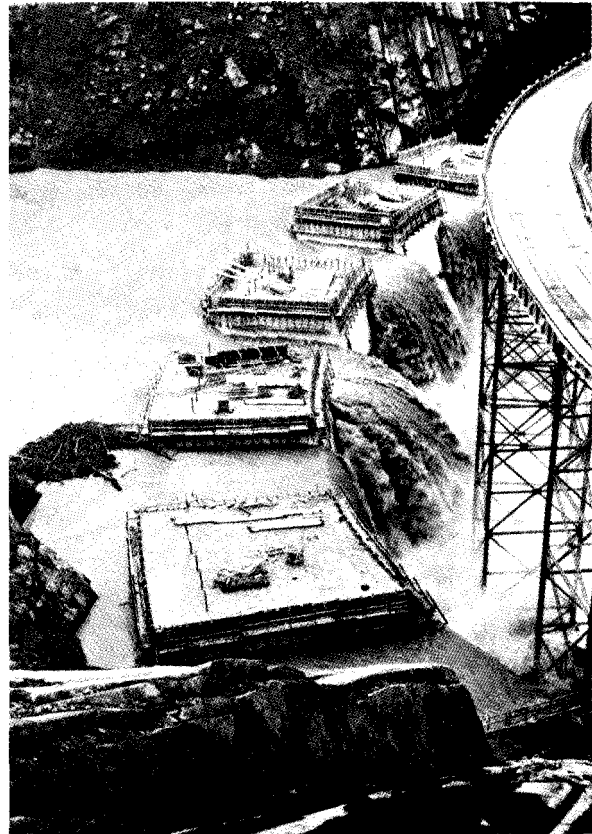
Figure 5-1. View from right abutment of partially completed Monticello Dam in California, showing water flowing over low blocks.-SO-1446-R2
