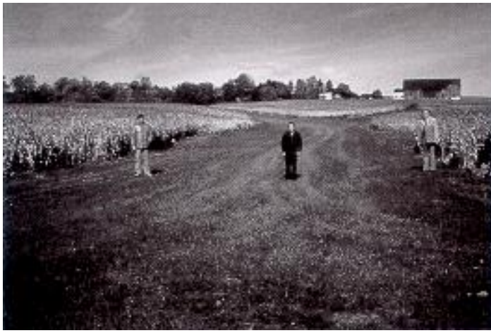
Figure 3. A properly constructed and maintained grassed waterway.
