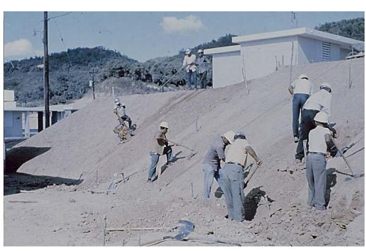
Soil erosion occurs when the soil surface is exposed to rain or runoff. Unprotected soil particles are first dislodged by the impact of raindrops or surface runoff. These loosened particles may then be moved by stormwater and deposited as sediment at some downstream location.
