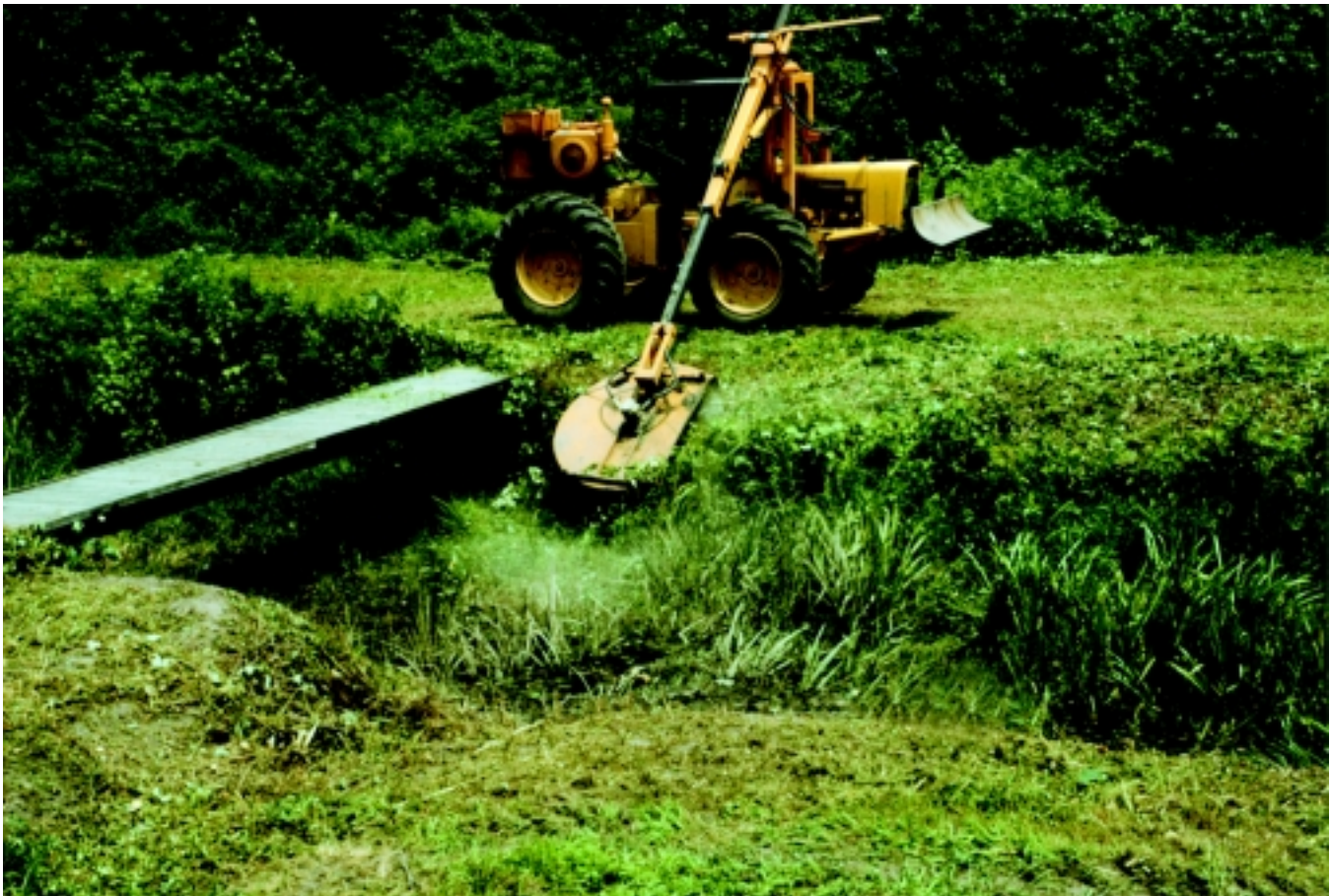
Figure 14–20 Maintenance by mowing
