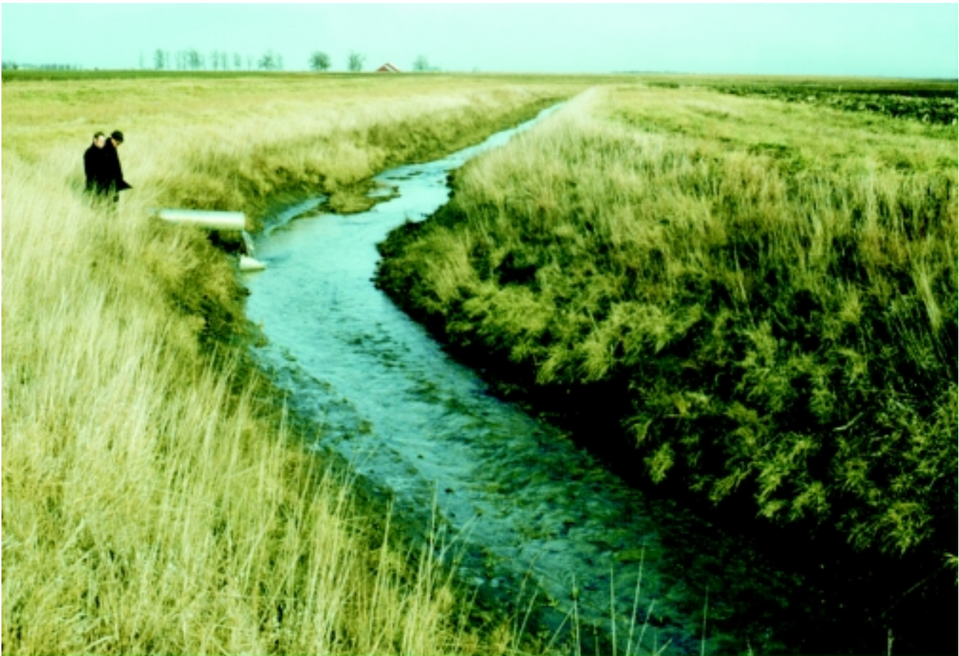
Figure 14–18 Main drain with spoil banks spread
