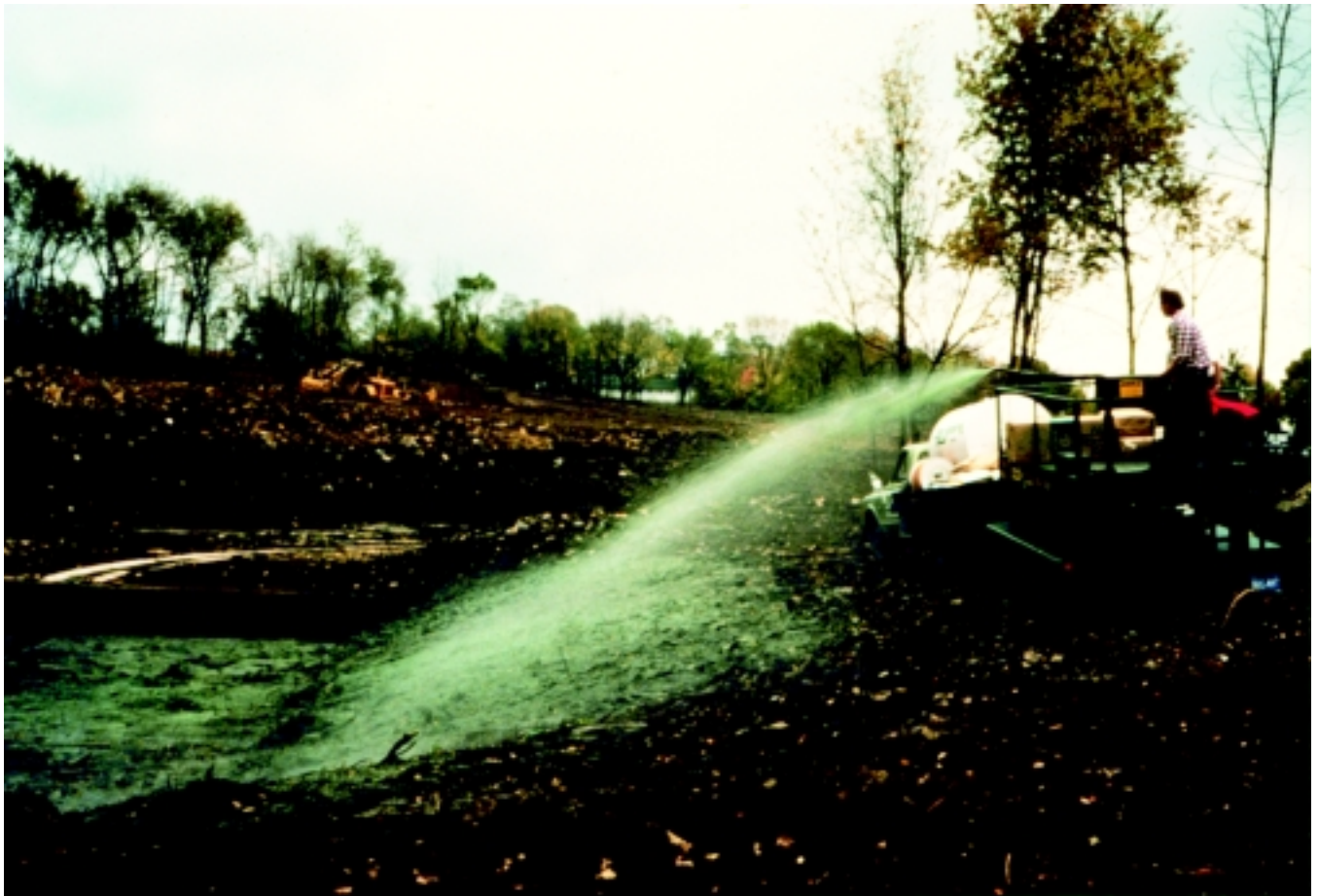
Figure 14-19 Seeding newly constructed drain
