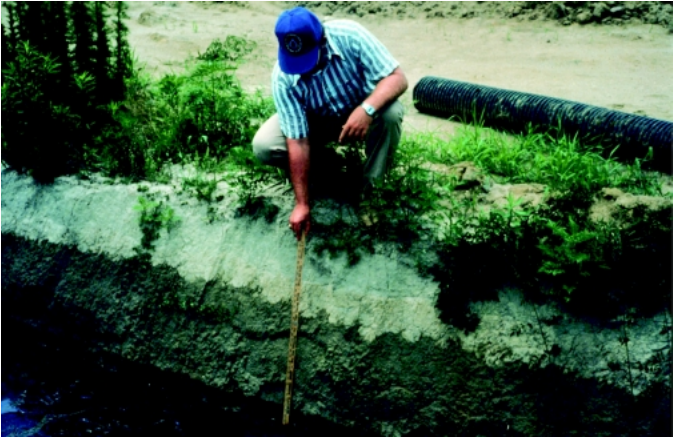
Figure 14-59 Monitoring water table depth
