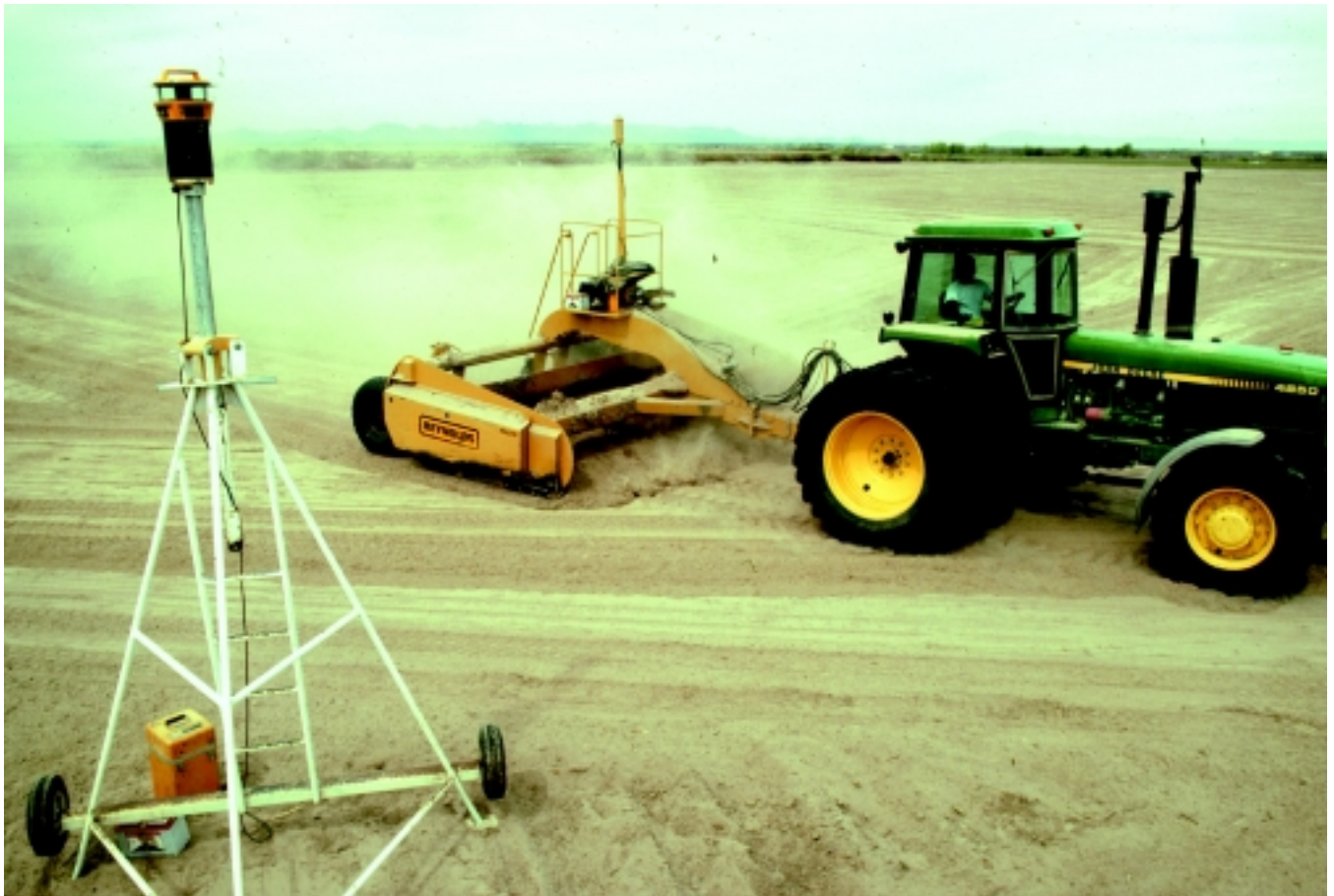
Figure 14-9 Earthmoving scraper with laser grade control
