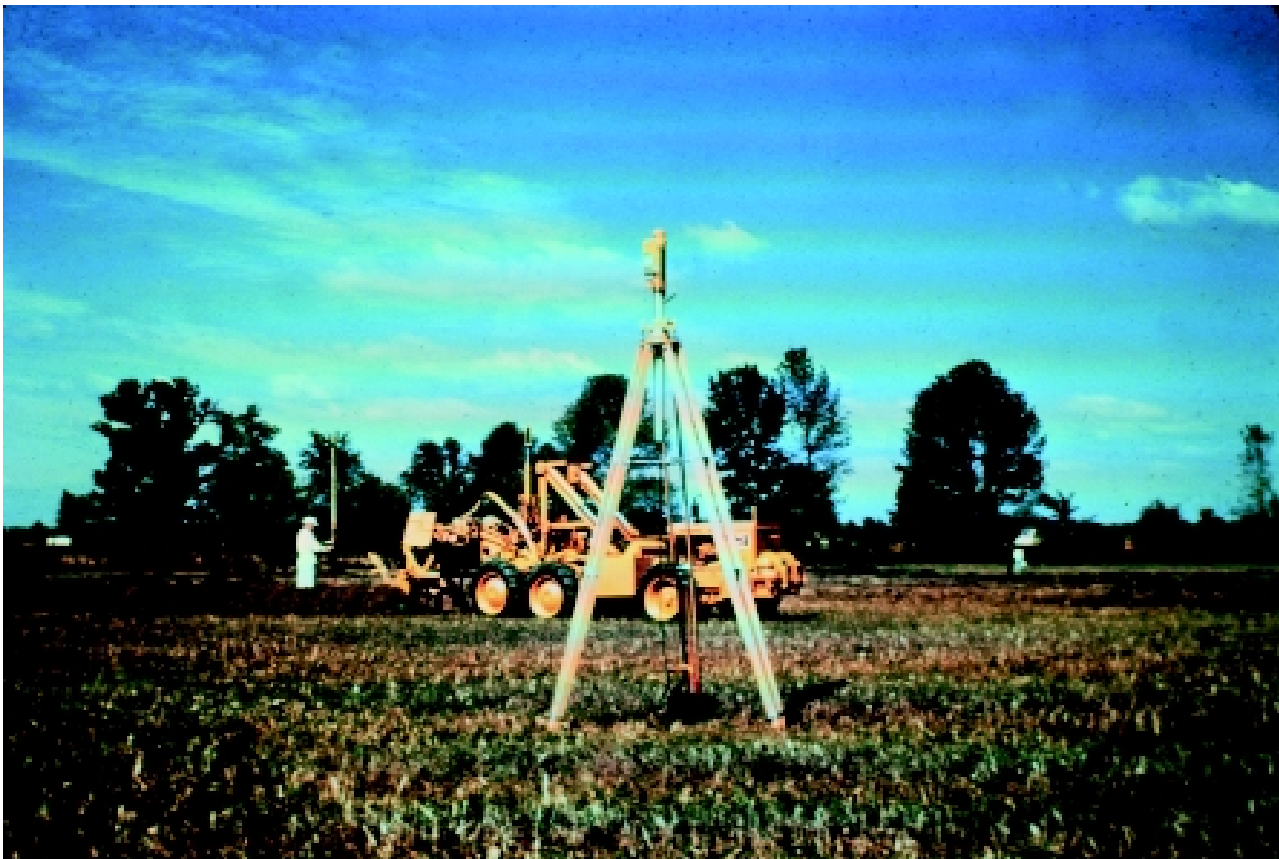
Figure 14-45 Laser grade control
