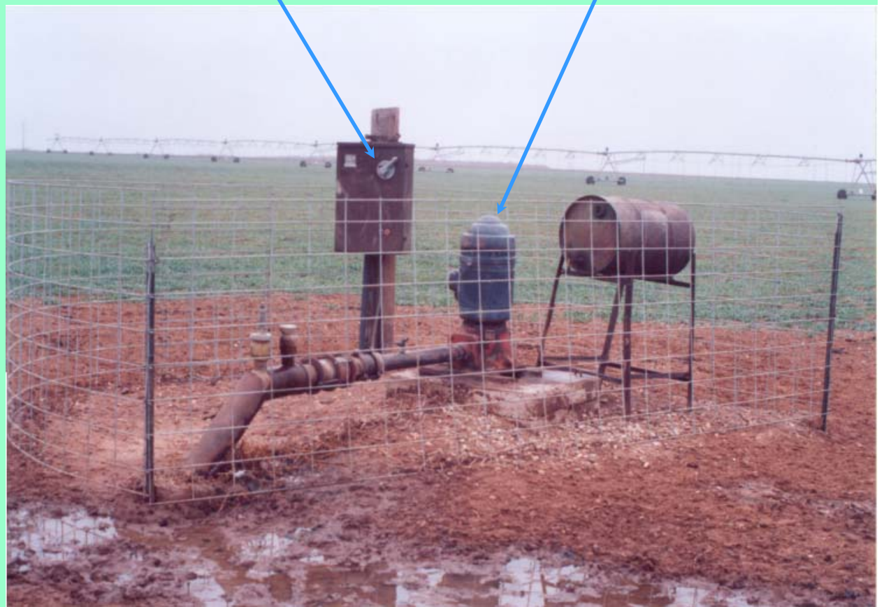
Pump Disconnect Switch
