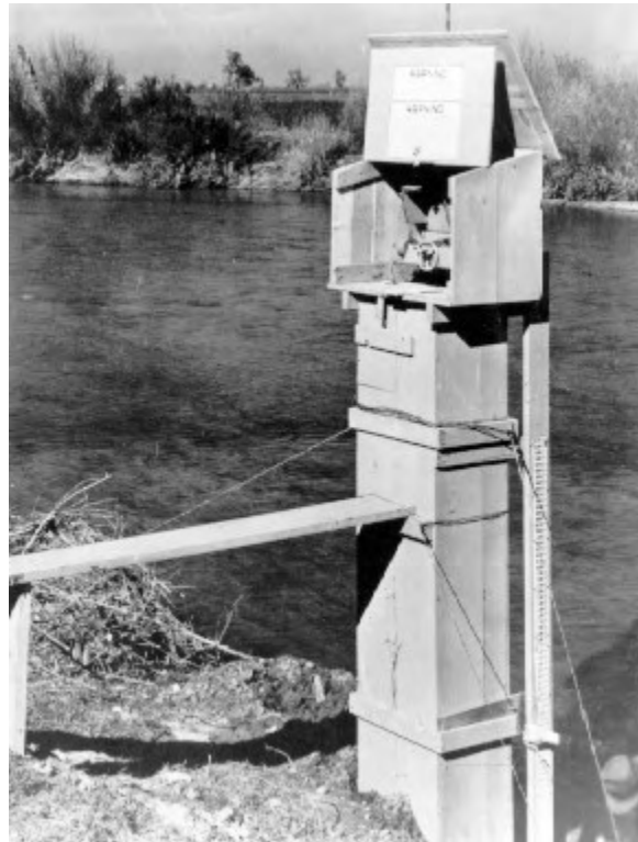
Figure 6-9 -- Stilling well and recorder house made of wood.
