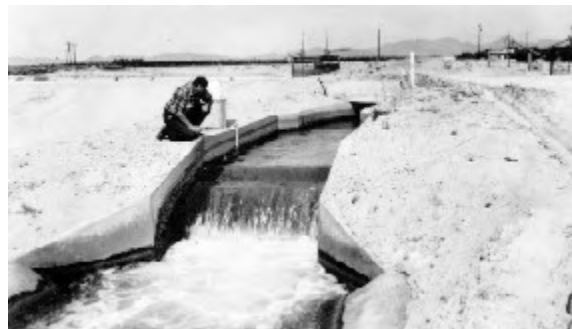
Figure 7-3 -- Suppressed rectangular weir at a canal drop.
