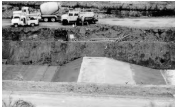
(a) Long-throated flume (broad-crested weir) under construction.
