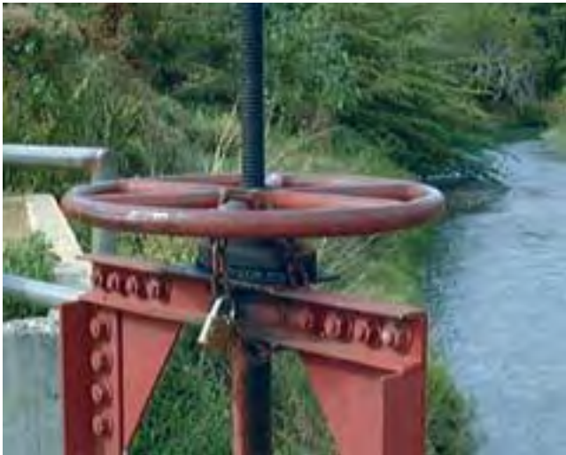
(a) Typical gate structure
