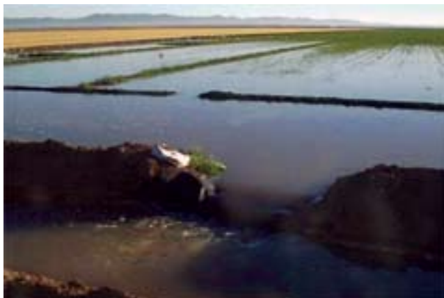
Figure 4–8 Tailwater outlet for a blocked-end border system
