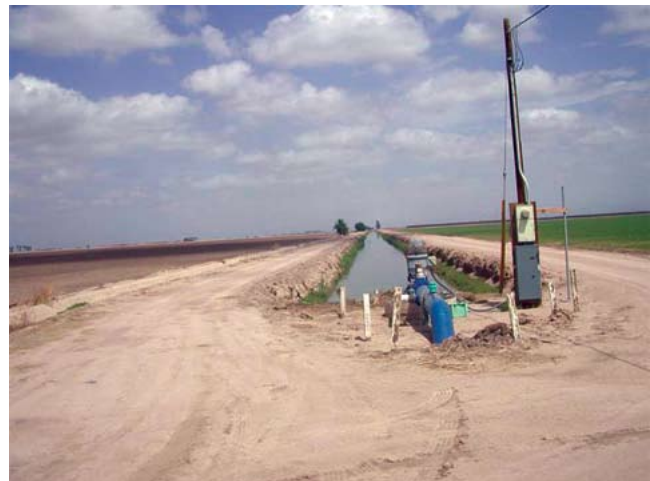
Figure 4-10 Typical tailwater recovery and reuse system
