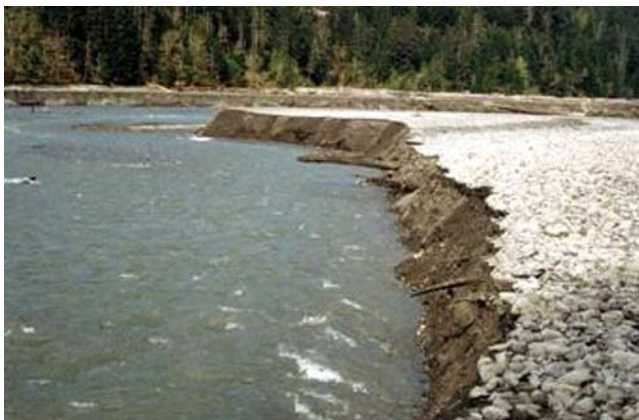
Figure 7-9 Degradation through armor layer
