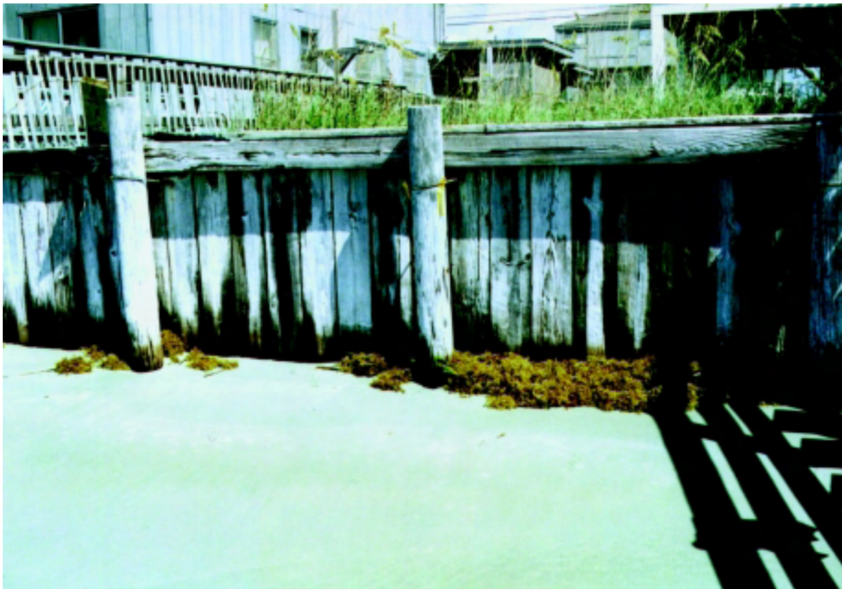
Figure 16–46 Timber bulkhead system
