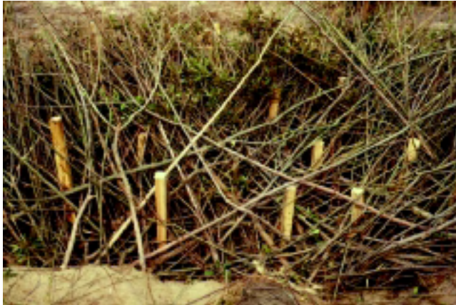
Figure 16–11a Live branches installed in criss-cross configuration (Robbin B. Sotir & Associates photo)
