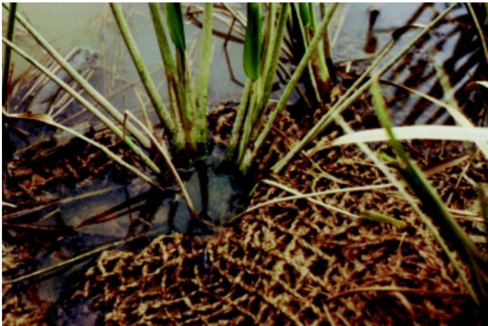
Figure 16–55c Established reed clump system (Robbin B. Sotir & Associates photo)
