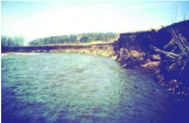
Figure 16–25a Pre-construction streambank conditions (Don Roseboom photo)
