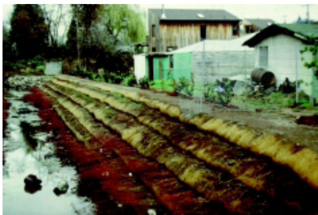
Figure 16–13b A vegetated geogrid immediately after installation (Robbin B. Sotir & Associates photo)
