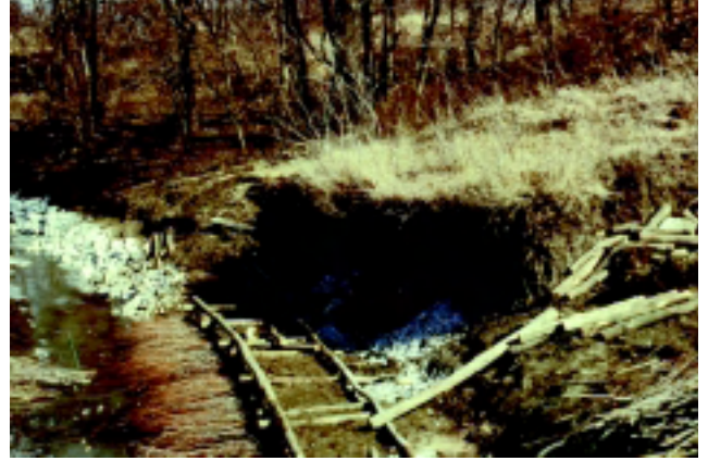
Figure 16-15b A live cribwall during installation
