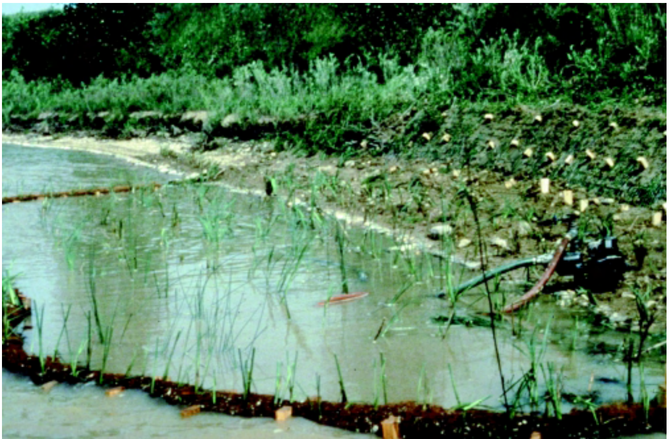
Figure 16-57 Coconut fiber roll system
