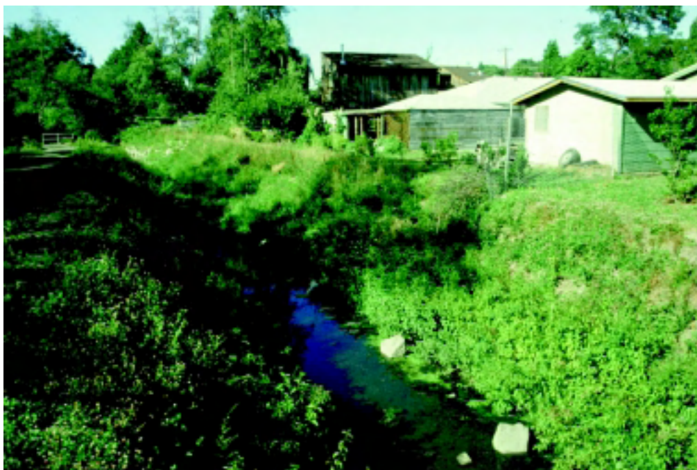
Figure 16–13c Vegetated geogrid 2 years after installation (Robbin B. Sotir & Associates photo)
