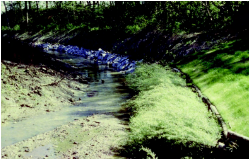
Figure 16-15c An established live cribwall system
