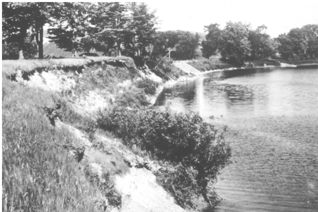
Figure 16-3a Eroding bank, Winooski River, Vermont, June 1938
