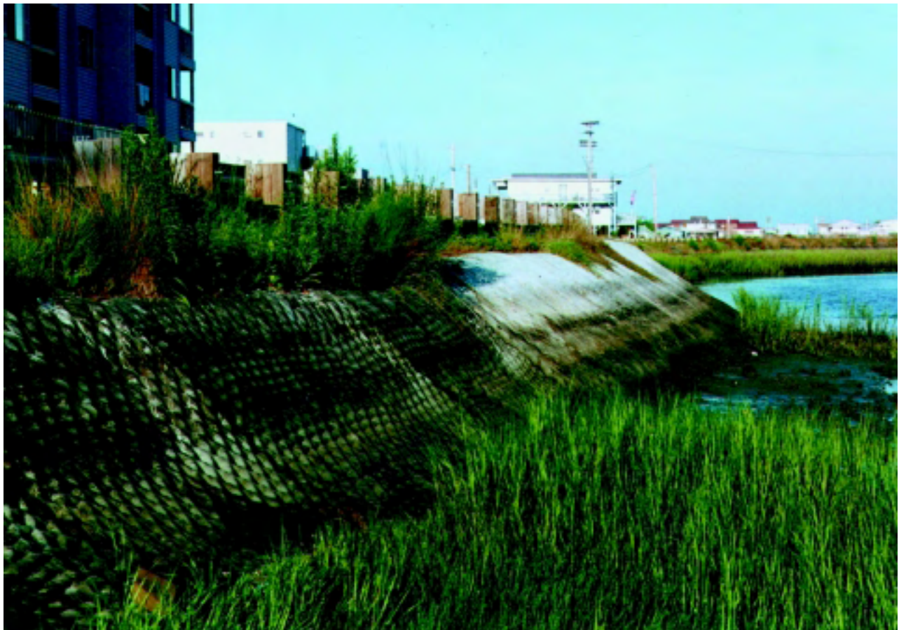
Figure 16–50 Concrete revetment (poured in place)
