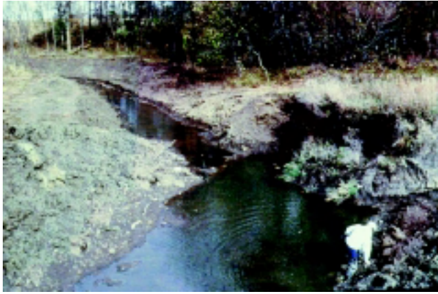
Figure 16-15a Pre-construction streambank conditions
