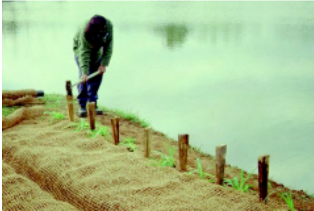
Figure 16–55a Installing dead stout stakes in reed clump system (Robbin B. Sotir & Associates photo)
