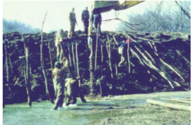
Figure 16–25b Installing dormant posts (Don Roseboom photo)
