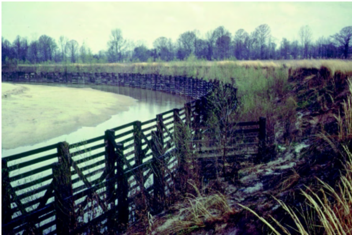
Figure 16–28 Slotted board fence system
