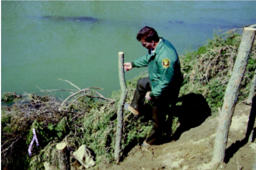
Figure 16–21a Tree revetment system with dormant posts
