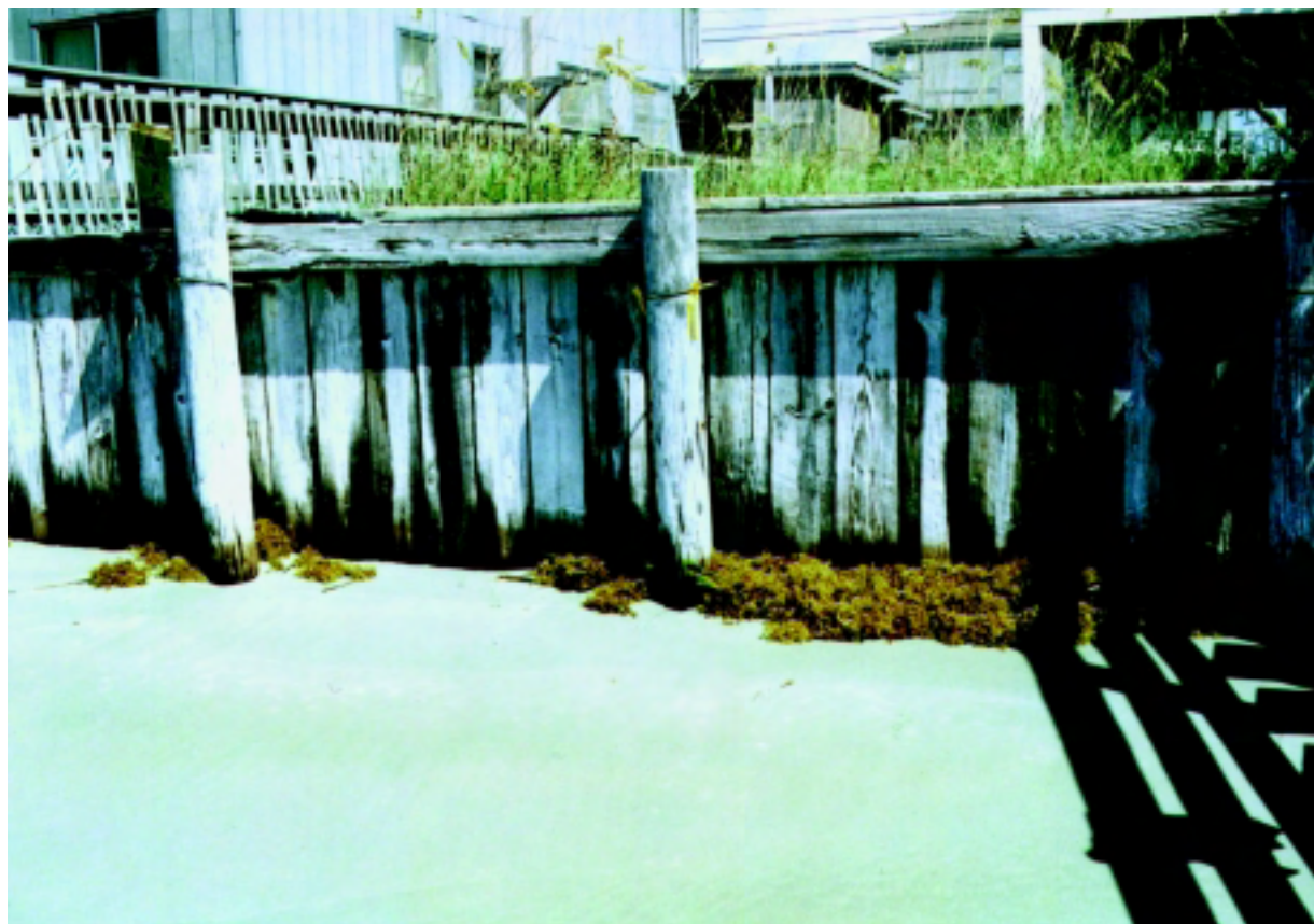
Figure 16–46 Timber bulkhead system
