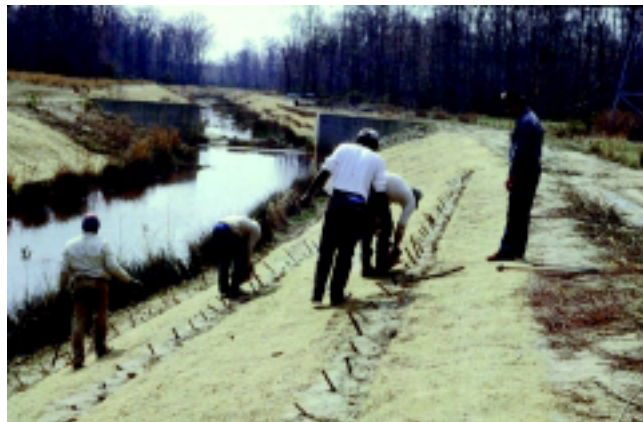
Figure 16–9b Installing live stakes in live fascine system (Robbin B. Sotir & Associates photo)
