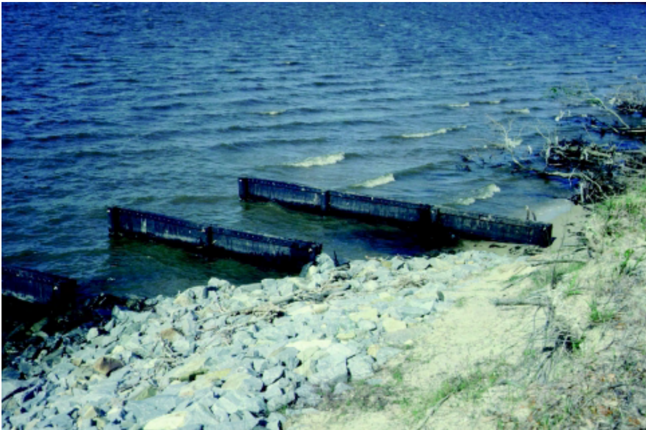
Figure 16–45 Timber groin system
