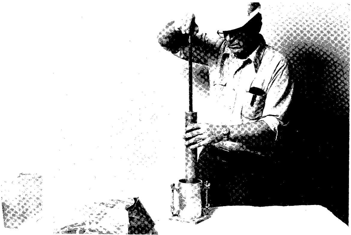
Figure 3-43—Compacting soil in the mold.
