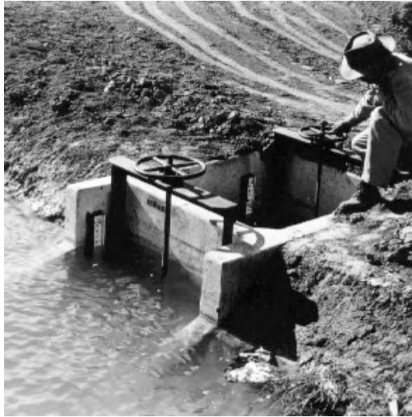
Figure 9-3 -- A single-barrel CHO turnout.
