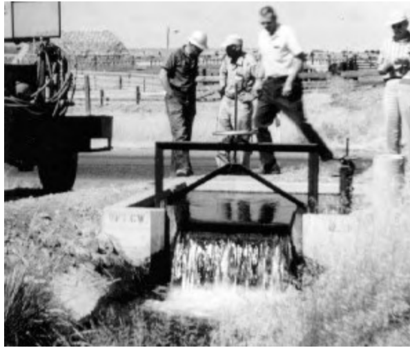
Figure 7-14 -- Adjustable Cipolletti weir in a division box.
