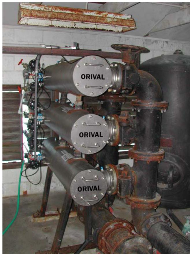
Figure 2. Three High Performance Stainless Steel Filters
