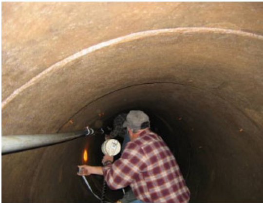
Figures 5 & 6: Photos show the installation into one of the TCCA sites. The photo at right shows the Argonaut-SW cradled in a protective "shoe" that helps deflect debris away from the instrument
