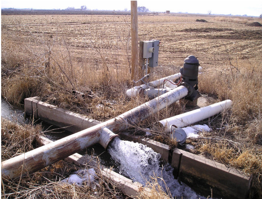
Fig. 3. Retiming well in operation. Water is pumped from the ground and is delivered to the river to cover stream depletions from irrigation well pumping. Sometime in the near future, stream depletions from the retiming well will occur in the river, and must be covered.
