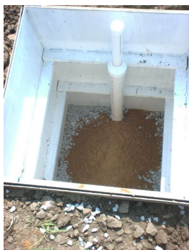
Figure 9. Install drain assembly, cover with gravel, sand.
