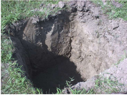
Figure 4. Remove soil and ensure bottom is level.
