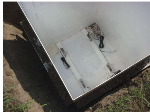
Figure 7. Install loadcells in outer tank.
