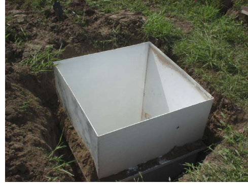
Figure 6. Backfill soil around outer tank.
