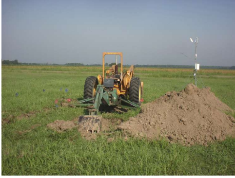
Figure 3. Choose location and begin excavation.
