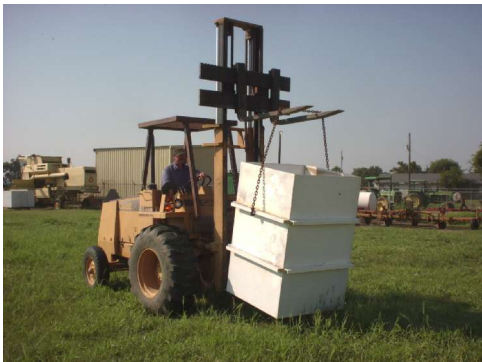
Figure 5. Install outer tank in hole.
