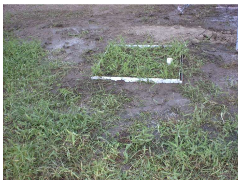
Figure 10. Backfill soil in inner tank.
