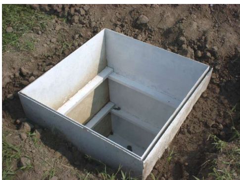
Figure 8. Install inner tank.
