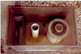
A roof washer may also be constructed or purchased that uses serviceable filters to eliminate debris. These require maintenance and cost between \$300 and \$600. They are not necessary for non-potable landscape watering systems.
