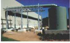
Steel fabricated tanks can be ordered through manufacturers. These need to be painted to enhance longevity.
