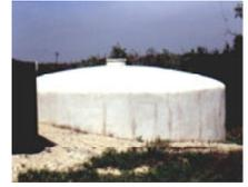
Stone tanks are very expensive to build correctly, but were the method of choice years ago. They can be difficult to repair and maintain.
