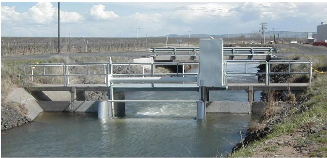
**Figure 4. This check structure is controlled by a Langemann gate and control is integrated with a SCADA system. Langemann gates function as a check structure and can be used for flow measurements.**
