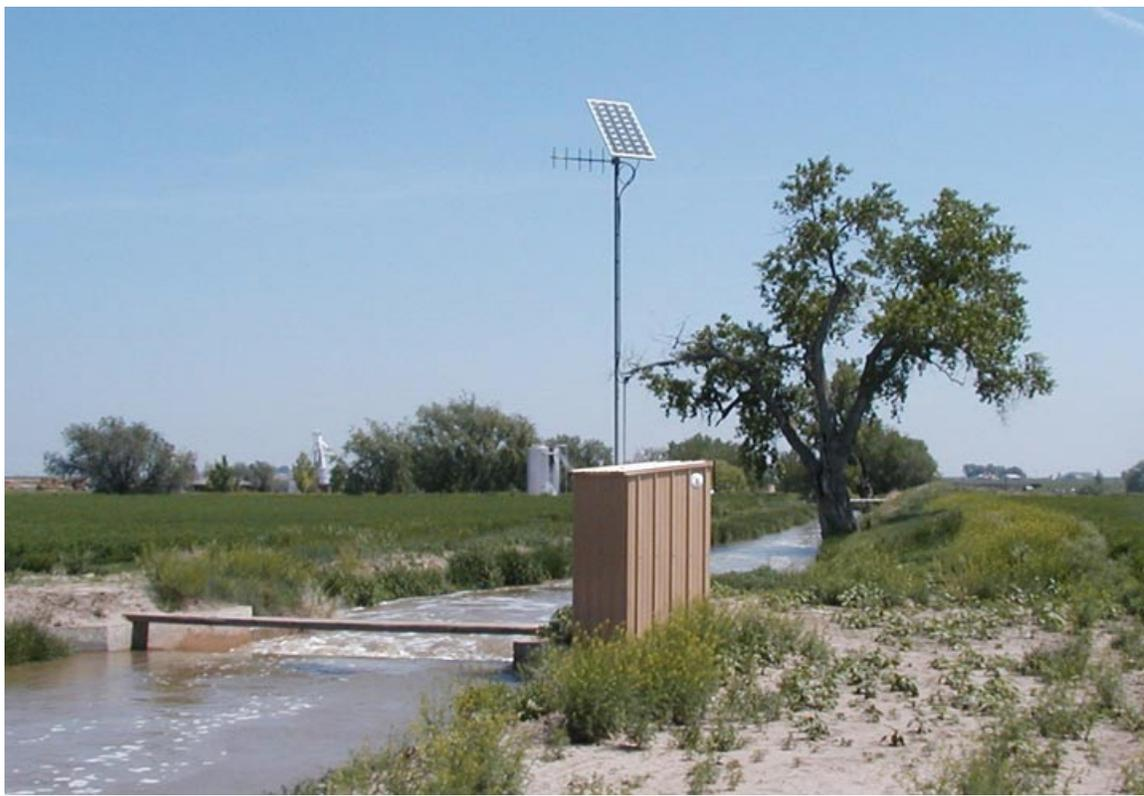
**Figure 1. An example of a rated canal section which is remotely monitored using a SCADA system. RTU equipment is 12-volt DC powered from a solar panel that maintains a charge on a battery. Communication with the site is via radio.**
