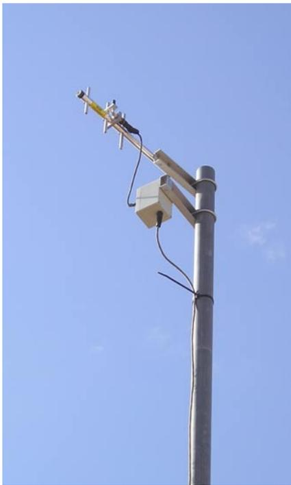
**Figure 5. The SCADA system at Central Arizona Irrigation and Drainage District (CAIDD) uses spread spectrum radio which is a relatively new type of radio system that does not require federal licensing. The spread spectrum radio is housed in the white enclosure and the directional antenna shown has a line-of-sight range of approximately 5 miles. The antenna is mounted on a 2-inch galvanized steel pipe.**
