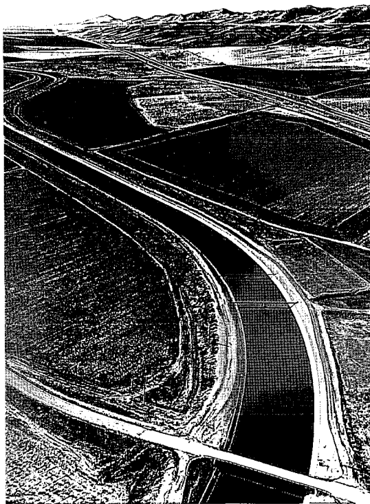
The California Aqueduct, above, as it meanders south along Interstate 5 near the Coast Range. The aqueduct delivers water 444 miles from the Delta to the city of Los Angeles, right.
