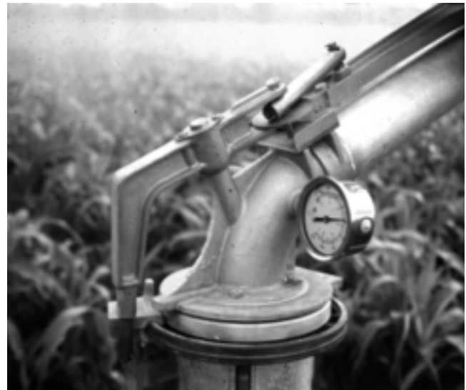
Figure 8. Pressure gauge installed on a traveling gun.
