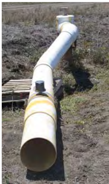
Figure 2. Designated pipe section for a propeller flow meter.
