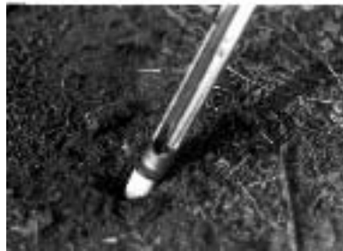
Figure 3. Block installation using a soil probe
