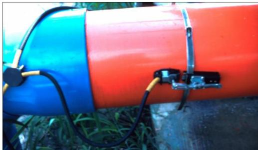
**Figure 7.** Transducers for ultrasonic flowmeter attached to 10-inch irrigation pipe
