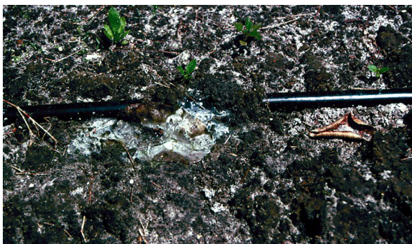
Figure 2. Drip emitter covered with sulfur slime that was blocking irrigation flow. Credits: Brian Boman UF/IFAS
