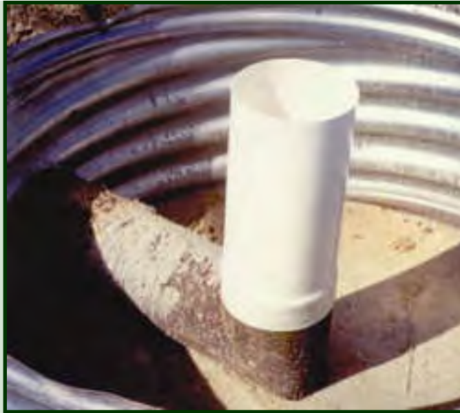
Riser pipe construction. Click on image to enlarge.
