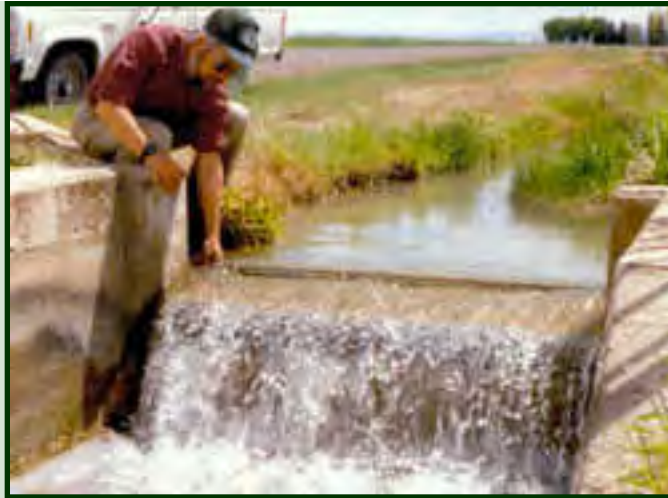
Angle iron turbulence bar increases turbulence in the flow. Click on image to enlarge.
