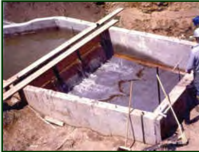
Large Overfall Screen at the sump inlet for several center pivot systems. Click on image to enlarge.
