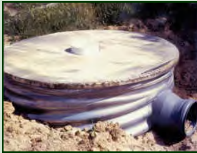
Bubbler Screen construction. Click on image to enlarge.
