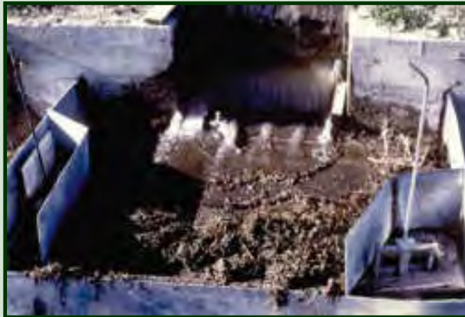
Horizontal Overflow Screens can be placed below canal gates. Click on image to enlarge.
