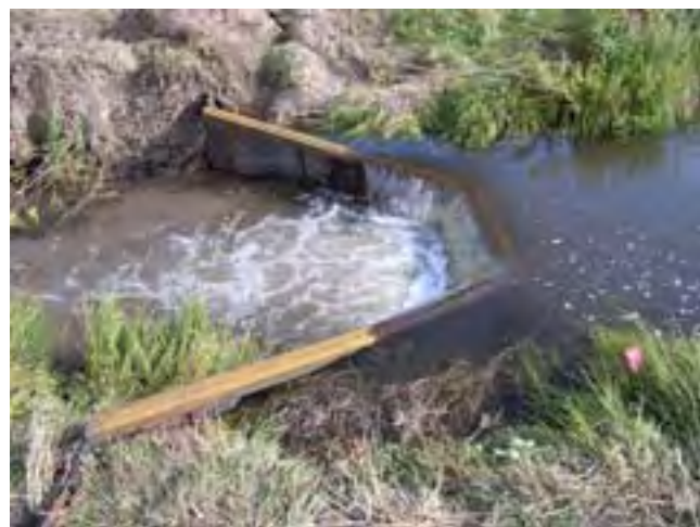
Figure 10 Sheet pile cross vane structure
