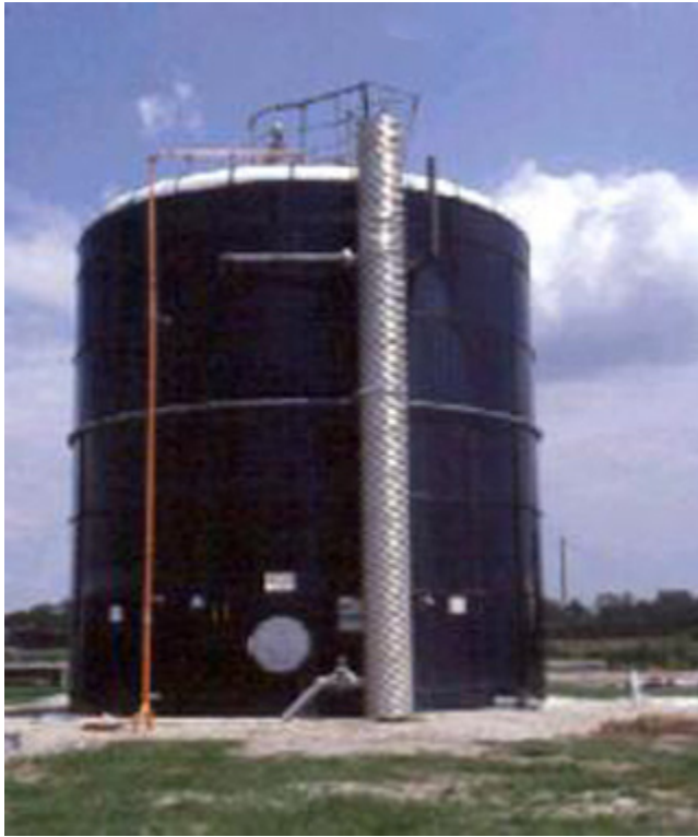
Figure 9 Fixed-film digester
