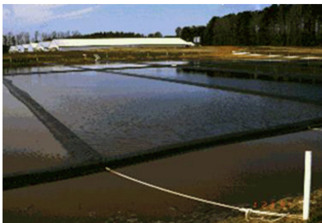
Figure 6 Partially covered anaerobic swine lagoon
