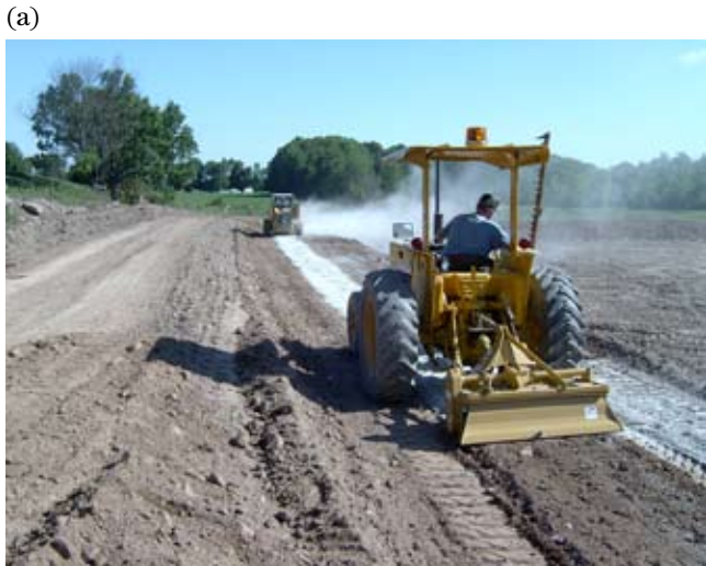
Figure 10D–8 Stair step method (photo credit John Zaginaylo, PA, NRCS)
