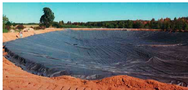
Figure 10D–2 Agricultural waste storage facility lined with a geomembrane
