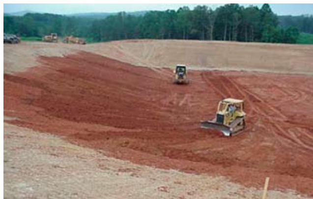
Figure 10D-7 Bathtub construction of clay liner (photo courtesy of NRCS Virginia)
