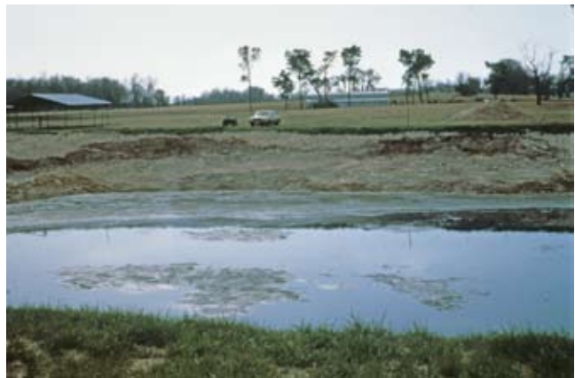
Figure 10D-17 Failure of compacted liner from uplift forces below clay blanket
