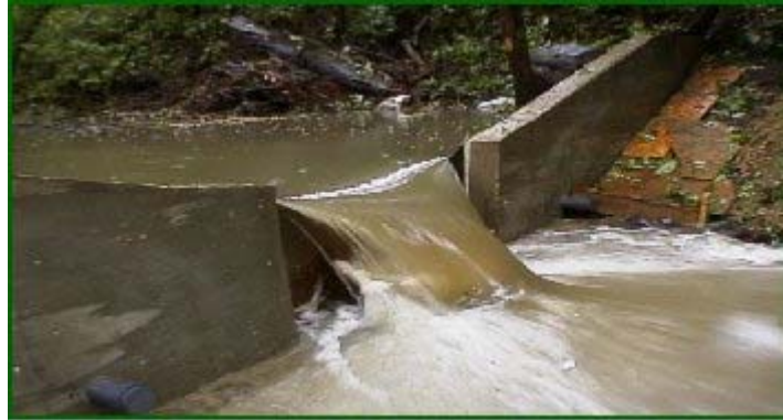
Figure 81. Sharp-crested weir in operation (USDA).
