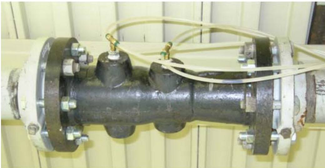
Figure 73. Venturi meter installed in a 4-inch pipeline, with manometer lines attached at the upstream end and at the throat of the meter.
