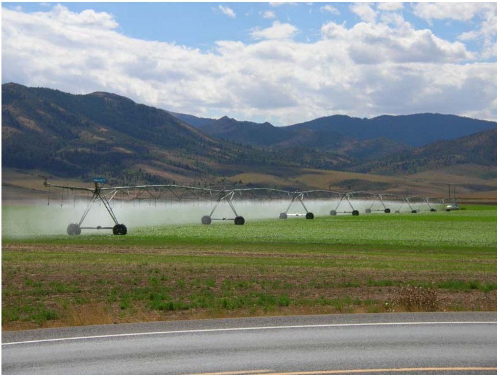
Figure 65. Central pivot irrigation system near Grace, Idaho.
