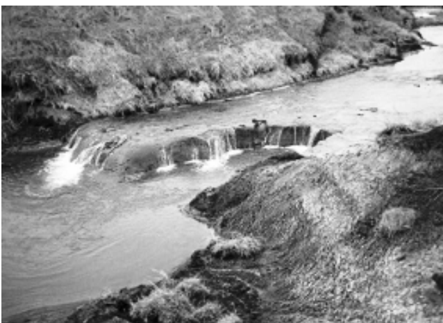
Figure TS3B-3 Nickpoint eroding headward
