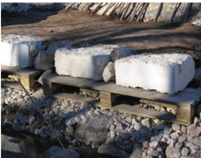
Figure TS14O-2 LUNKERS installed over a stone base
