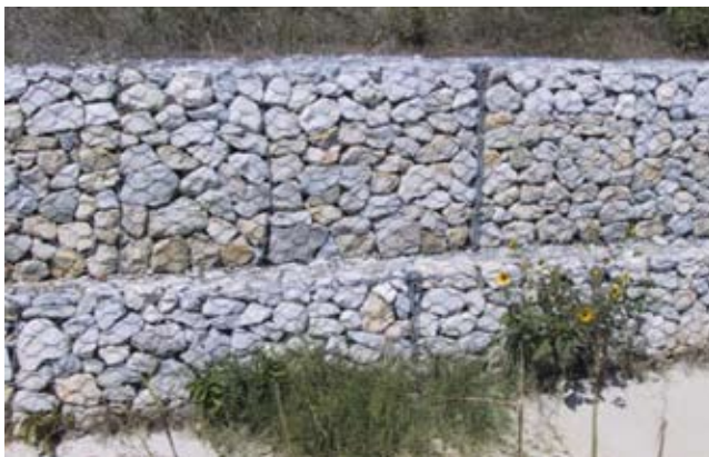
Figure TS14K-11 Gabions showing a neat, compact, placement of stone with a uniform appearance
