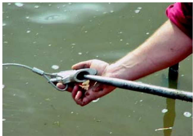
Figure TS14E-2 Drive rod being inserted into Duckbill ® anchor prior to installation
