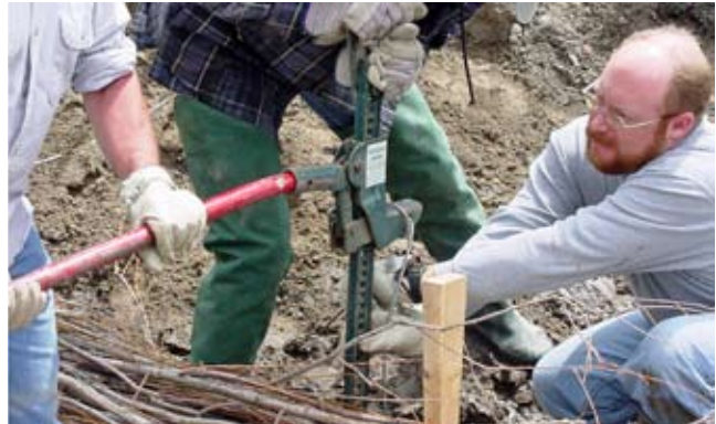
Figure TS14E-6 Hi-Lift ® jack being used to load-lock a Duckbill ® anchor
