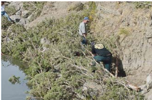
Figure TS14E-8 Boulders serve dual purpose: to stabilize the toe and secure brush revetment
