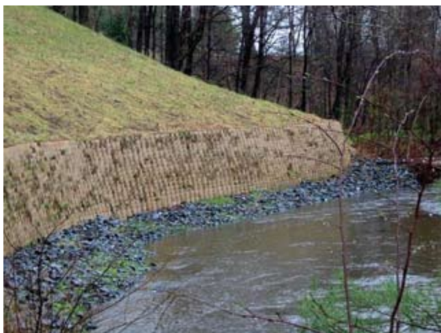
Figure TS14D-17 Geocell earth retaining structure (Photograph courtesy of Carl Gustafson, NRCS MA)
