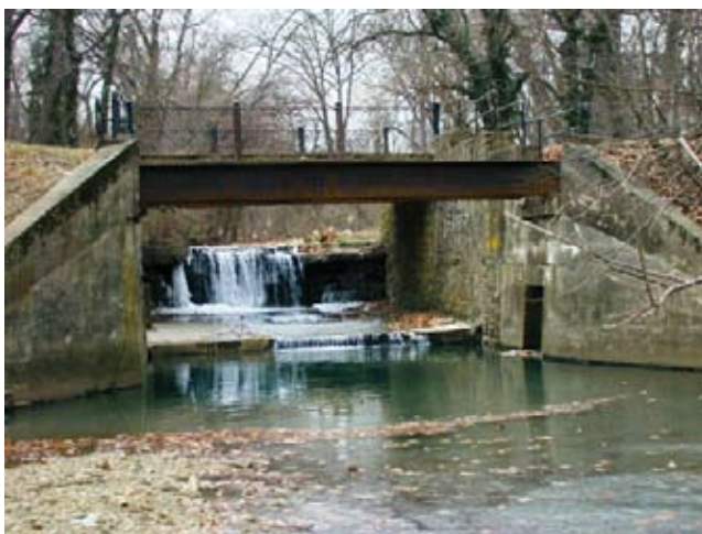
Figure 2-4 Fish blockage in stream
