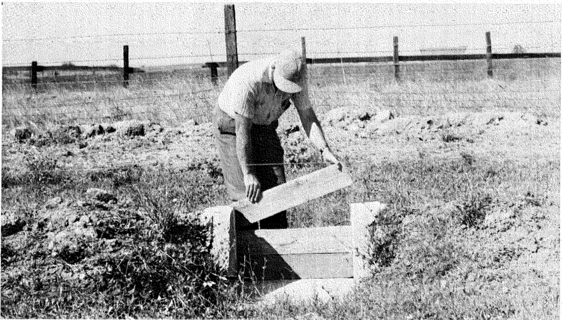
Figure 3-45.--Concrete turnout with a flashboard gate.
