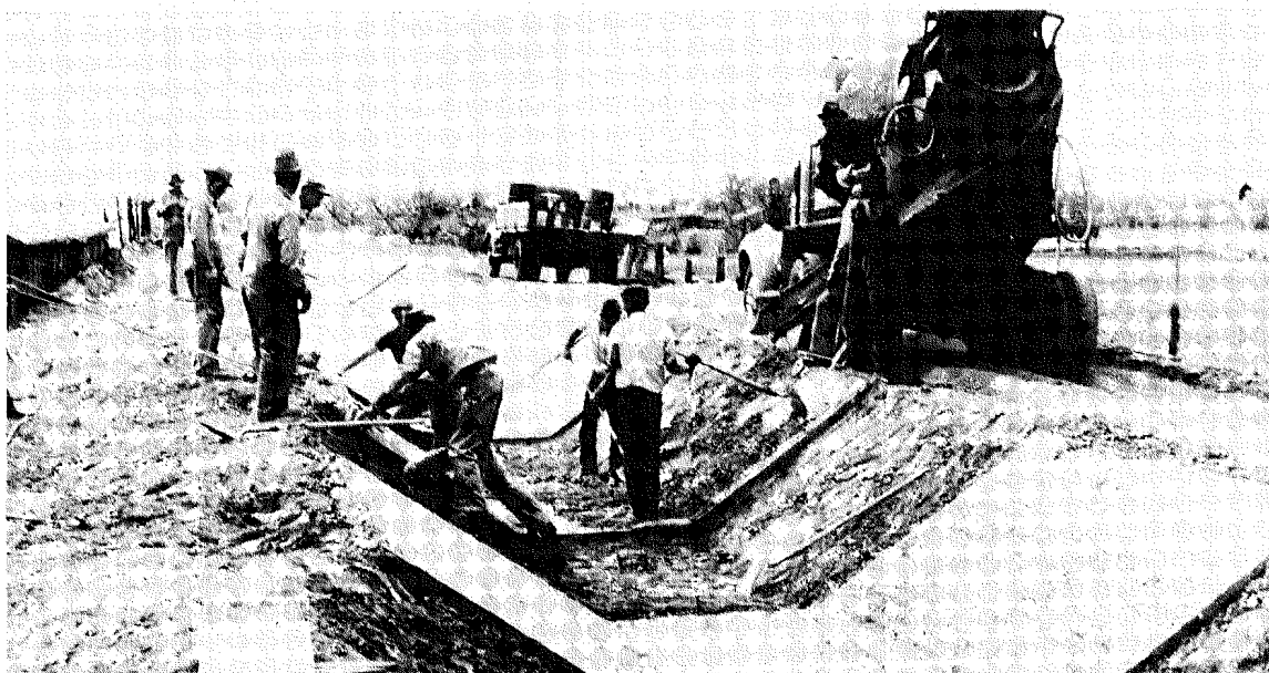
Figure 3-25.--Constructing concrete ditch lining by alternate-panel method.
