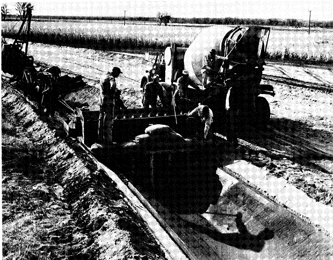
Figure 3-24.--Placing concrete ditch lining by slip-form method.
