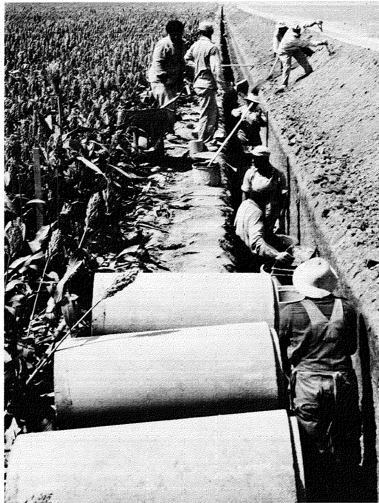
Figure 3-55.--Installing 15-inch concrete irrigation pipe.
