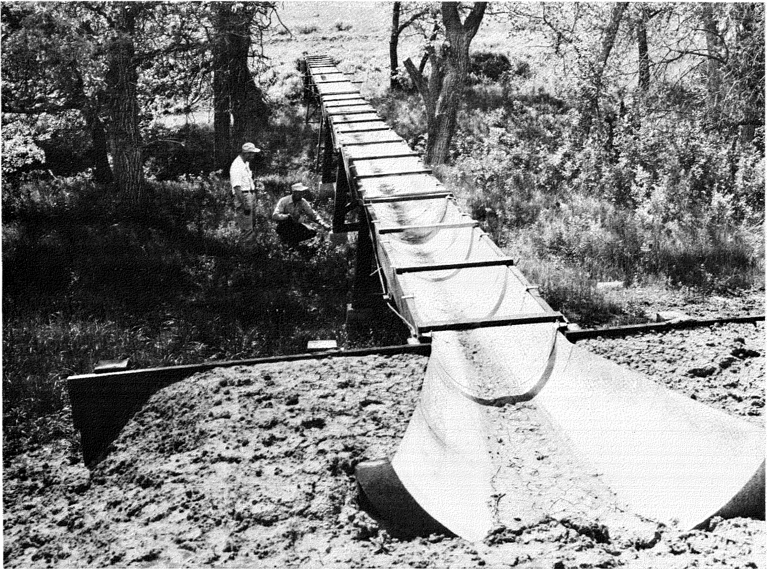
Figure 3-26.--Timber-supported metal flume.
