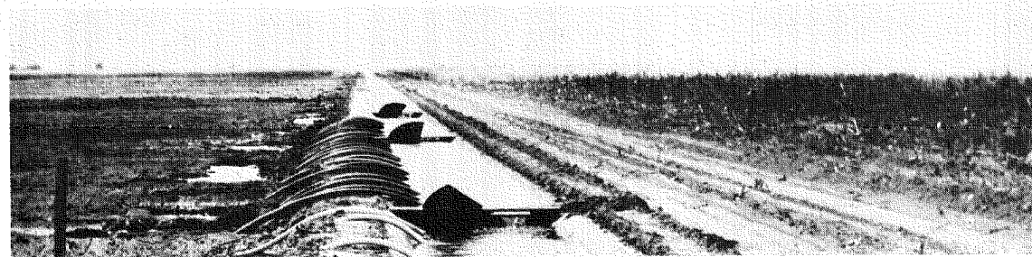
Figure 3-36.--Metal windless check.
