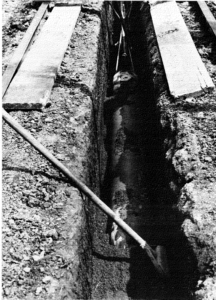
Figure 3-56.--Removing inside form from concrete pipeline cast in place.
